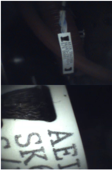
Fig. 16: Labeling behind equipment within rack and a close up view.
