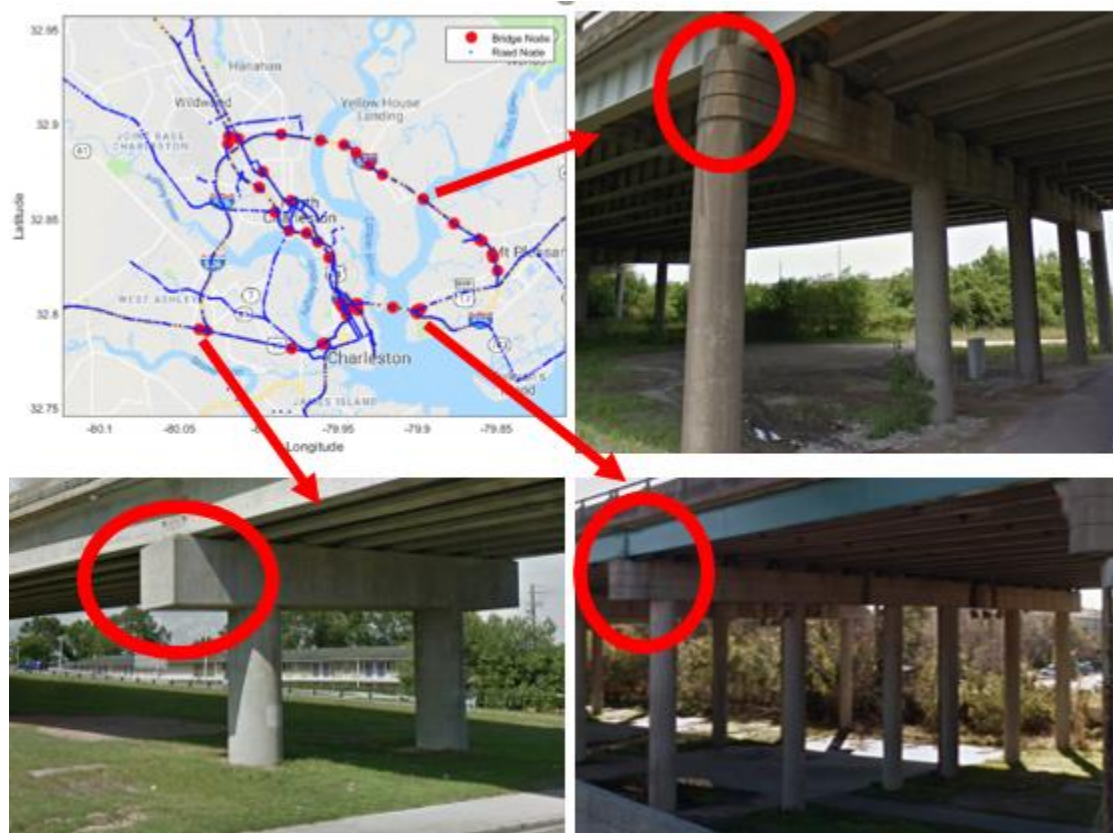
Figure 5.6: Examples of pile-to-bent cap connections
