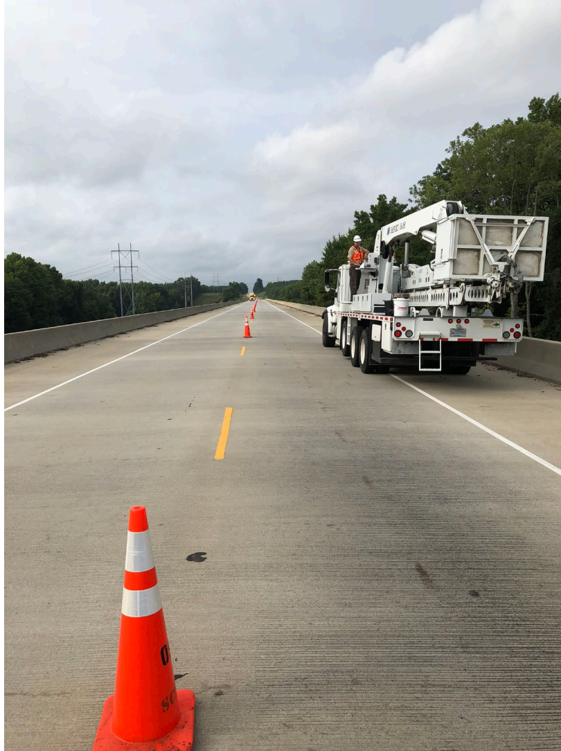
Figure 5.31: Lane closure of Bates Bridge.
