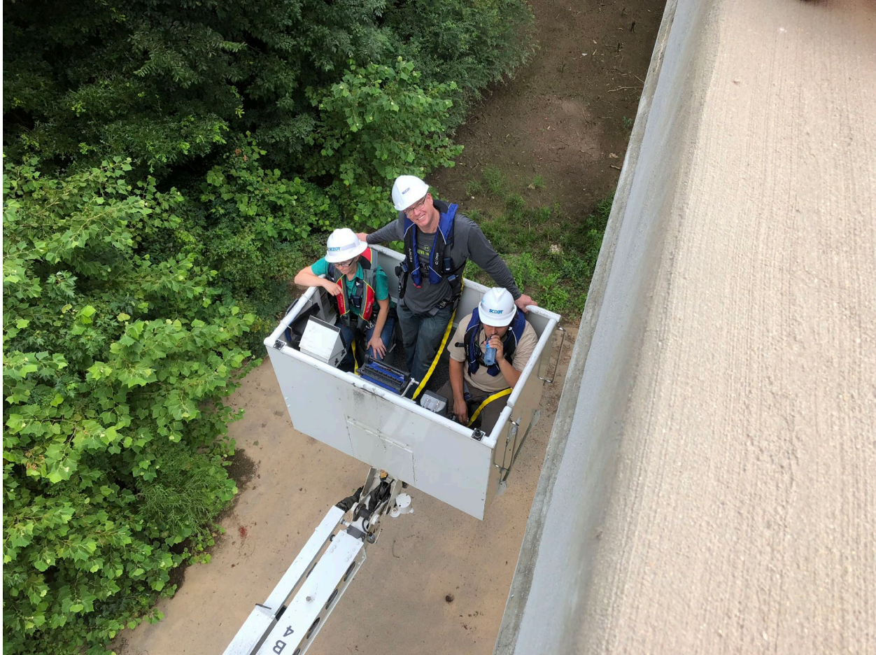
Figure 5.1: Traditional inspection with UBIT.
