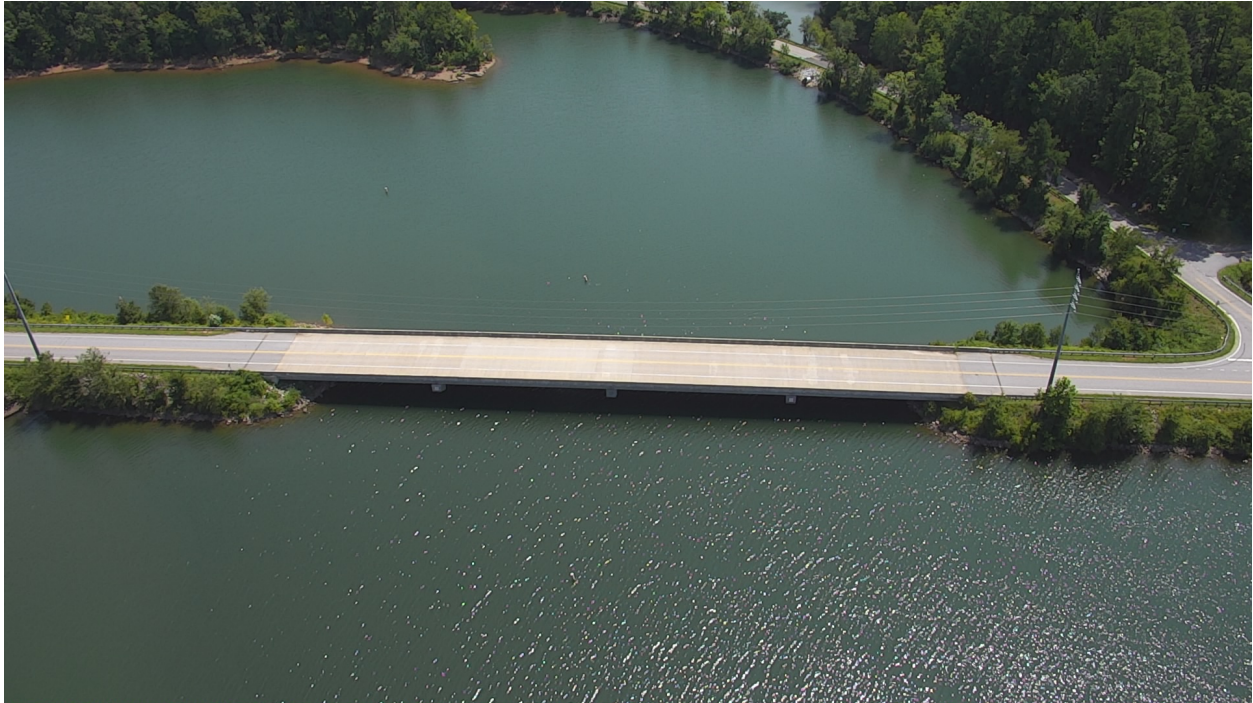
Figure 5.29: Remote test bridge #1.
