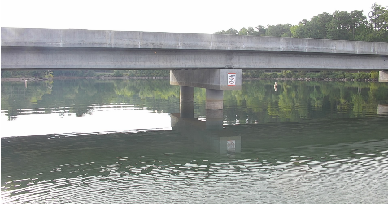
Figure 5.30: Remote test bridge #2.
