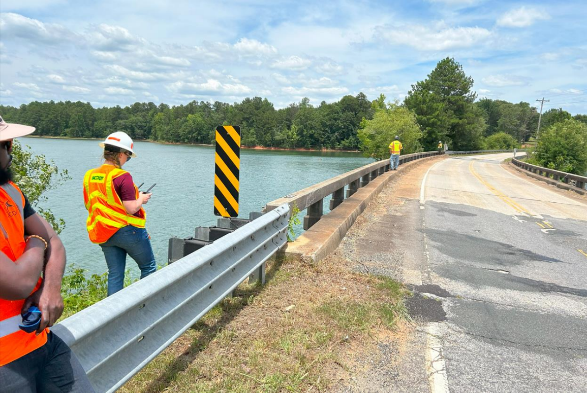
Figure 9: Bootcamp #1, Day 2, Seneca Creek Bridge
