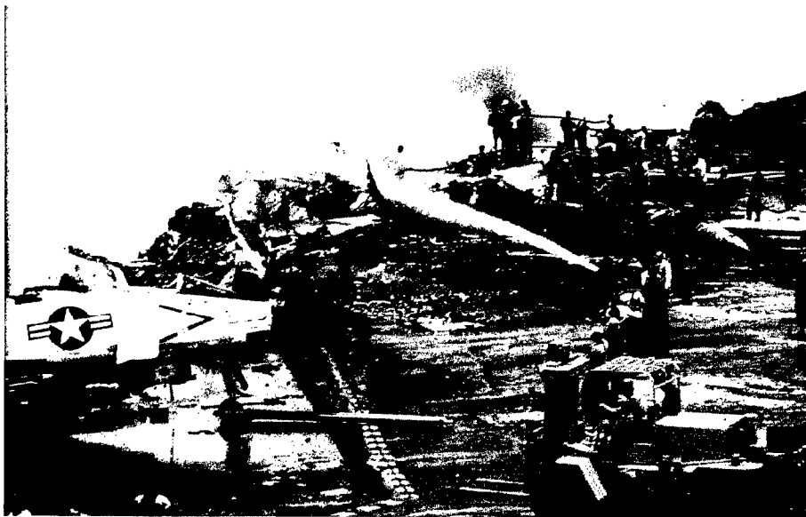
Figure 3. Aftermath of U.S.S. Forrestal EMI incident.
