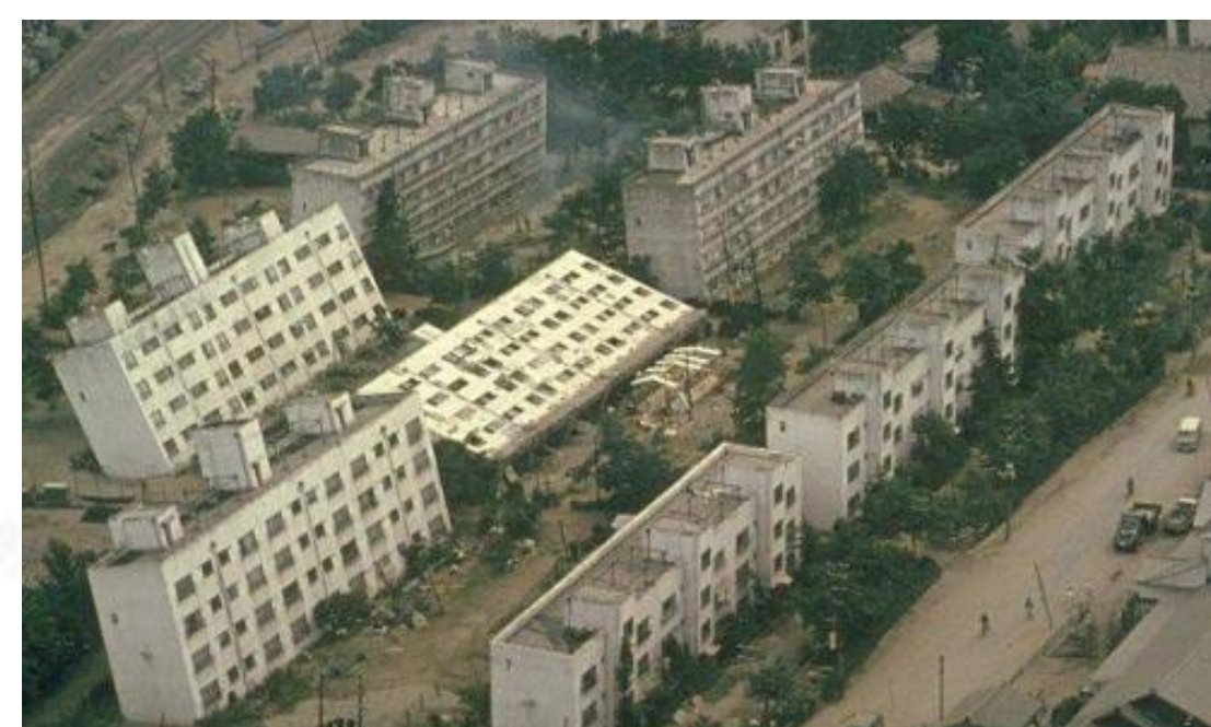
Figure 1. Soil liquefaction 1964 Niigata Earthquake
