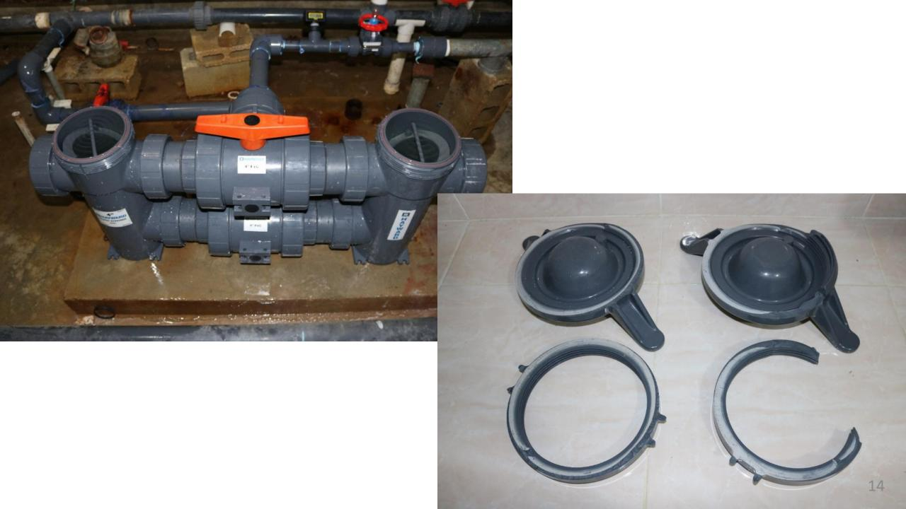
The most recently installed chlorinator is a tablet feeder built to handle the high system pressure (>100 psi).
