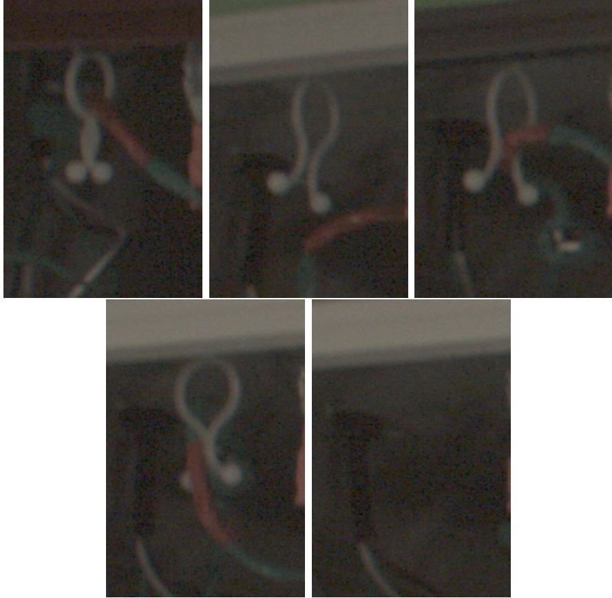
Figure 2.8: In the first figure, the wire harness is inside the wire holder (OK). Next, the wire holder is not tied and the wire is left dangling outside of the holder (NOK). Next, the holder is not tied and the wire can slip out (NOK). In the fourth figure, the wire is not going through the holder and in the last figure the holder is absent (NOKs).
