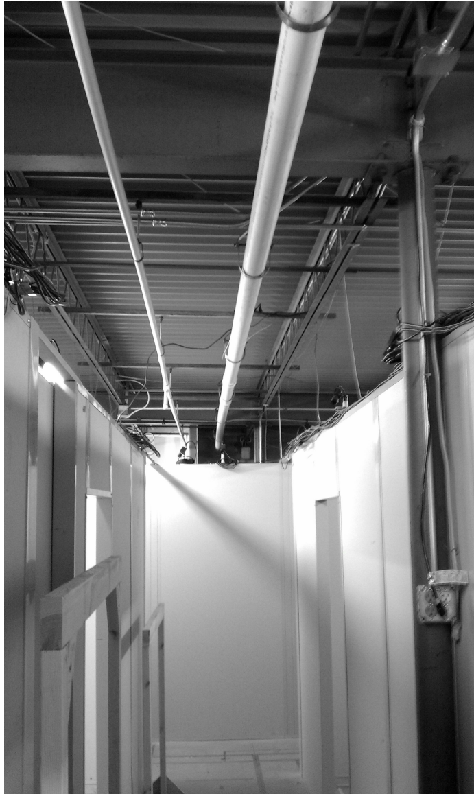
Figure 2.4: Photo of the Shoothouse facility's main hallway.
