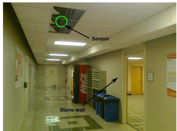
Figure 4 The facility and location of one of the eight sensors.
